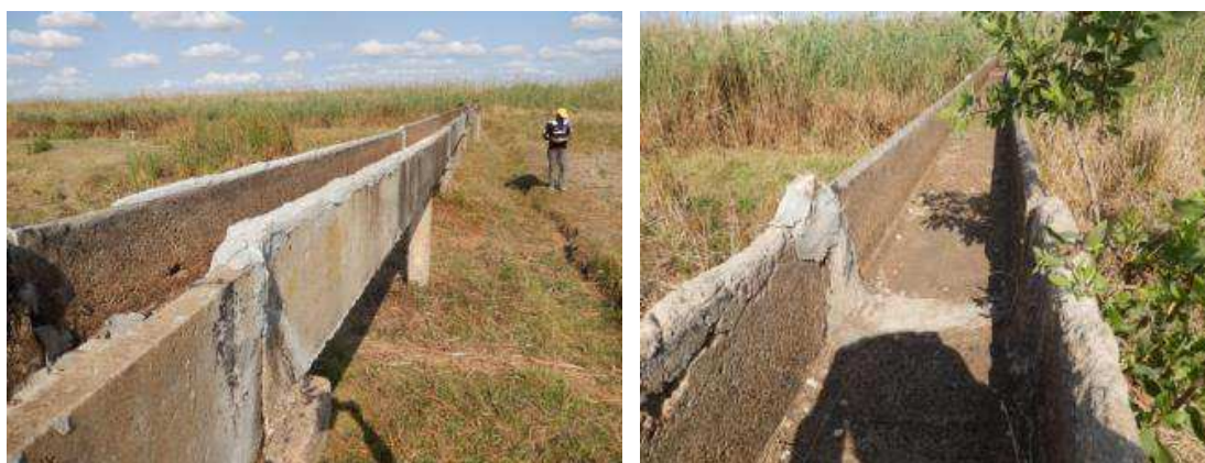
Photos 3.3: Minor repair by cement mortar
